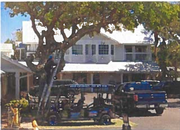
Existing Mixed-Use Building in Indian Rocks Beach
