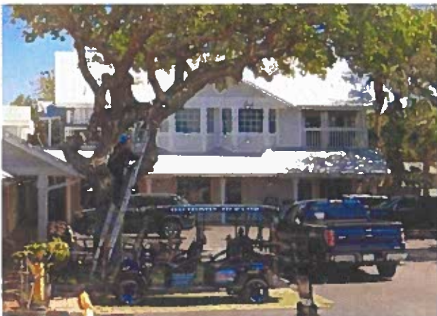
Existing Mixed-Use Building in Indian Rocks Beach
