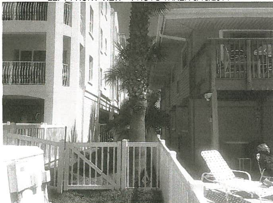
LEFT FRONT VIEW – PHOTO TAKEN 3/13/2014
