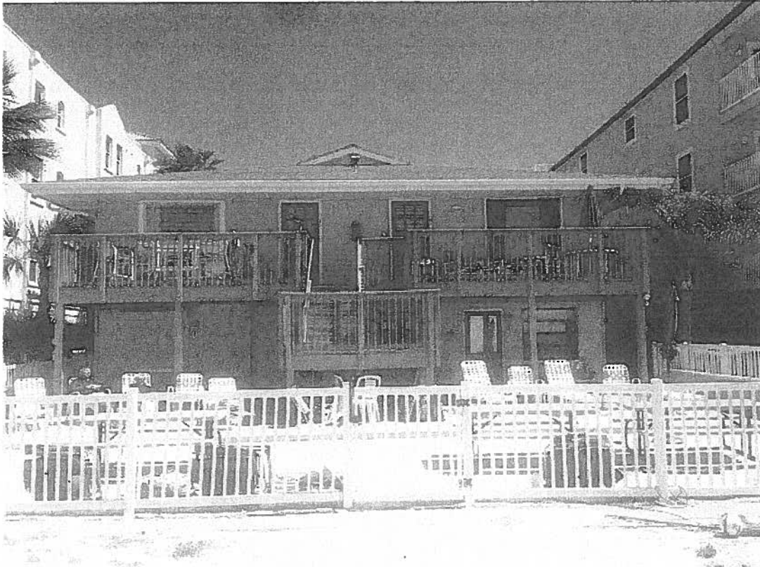
REAR VIEW – PHOTO TAKEN 3/13/2014
