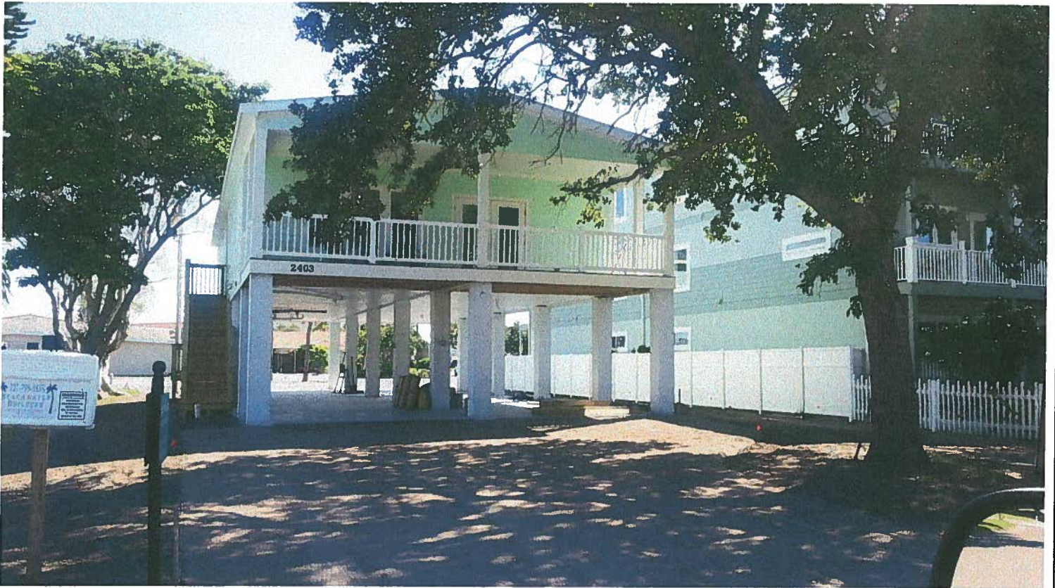
FRONT (WEST SIDE) TAKEN 10/23/2014
